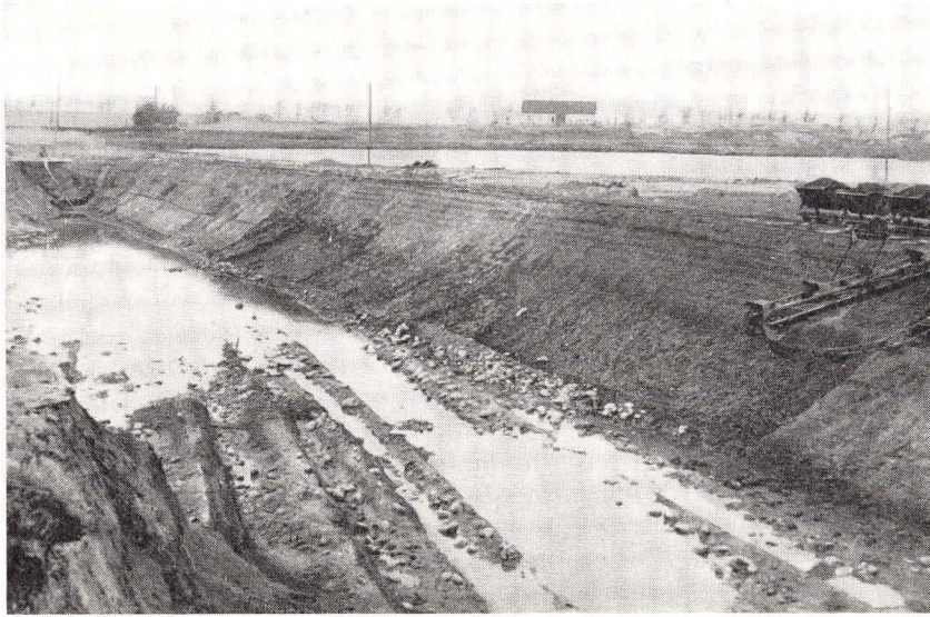
Fig. 58. The eastern clay pit of the brickworks of Måde. The north wall of the new zone, where digging was started about 1960. In the dark zone in the wall west of the middle, the sample of clay was taken the analysis of which is found in Table 49. On the right of this zone the somewhat paler moraine sand is seen. In the background the water-logged clay pit shown in fig. 55.
