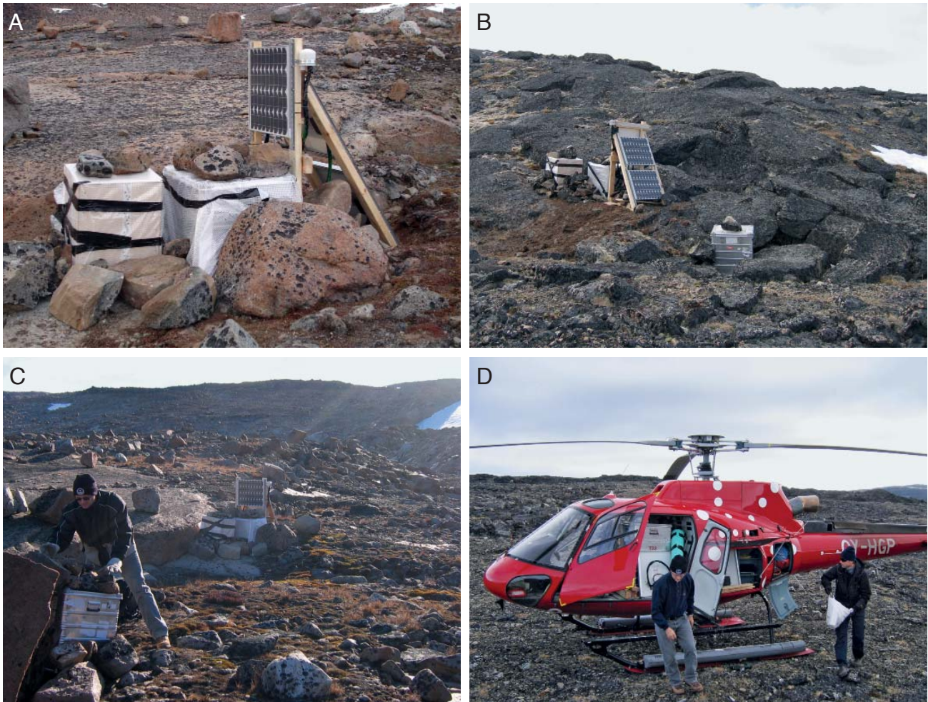
Fig. 2. The seismic stations. The almost 100 % exposure of bedrock allows for all stations to be placed on hard rock. A: SA1G. The completed installation in 2006 with solar panels facing south, the sensor placed on bedrock and insulated, and just as the datalogger, protected against the elements. Photo: K.K Sand. B: SA2G was installed in 2006. Photo: P.H.Voss. C: SA4G packed in 2007 for return. Photo: H. Rasmussen. D: From SA3G. The seismic stations were deployed and returned by an Air Greenland AS350. Photo: H. Rasmussen.
