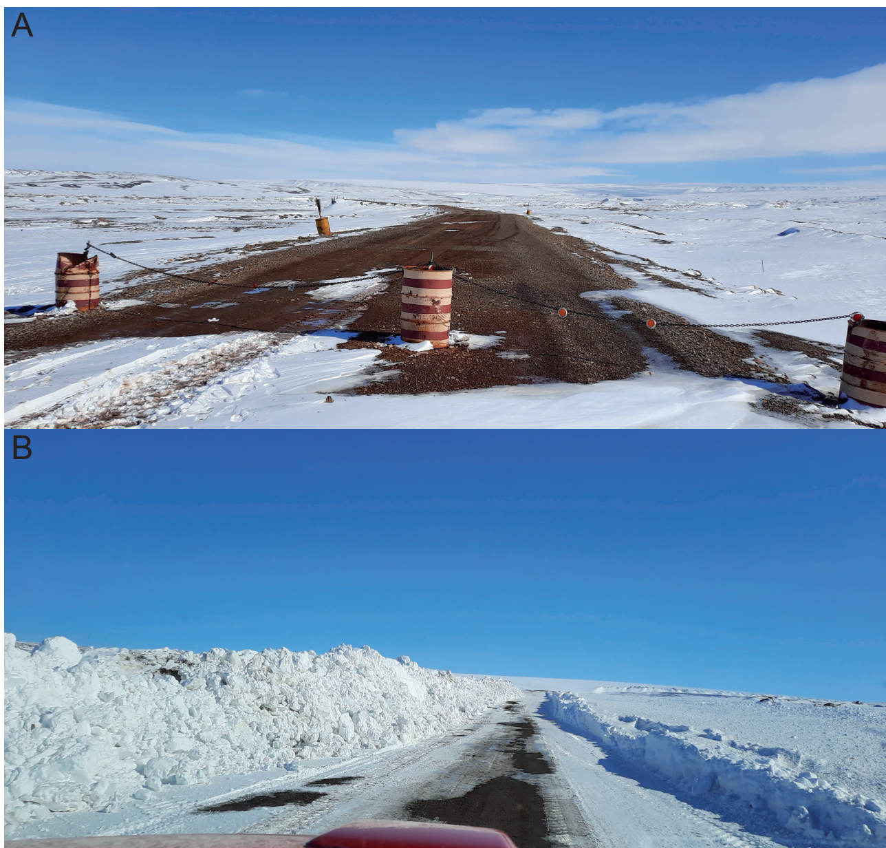
Fig. 8 View of the traverse. A: Photograph of a relatively elevated portion of the TUTO access road that remains snow-free in the spring (27 May 2023). Photo: William Colgan. B: Photograph of a relatively depressed portion of the TUTO access road where spring snow depth is >1 m (31 May 2023). Photo: William Colgan. The location of the photos is depicted in Fig. 2.
