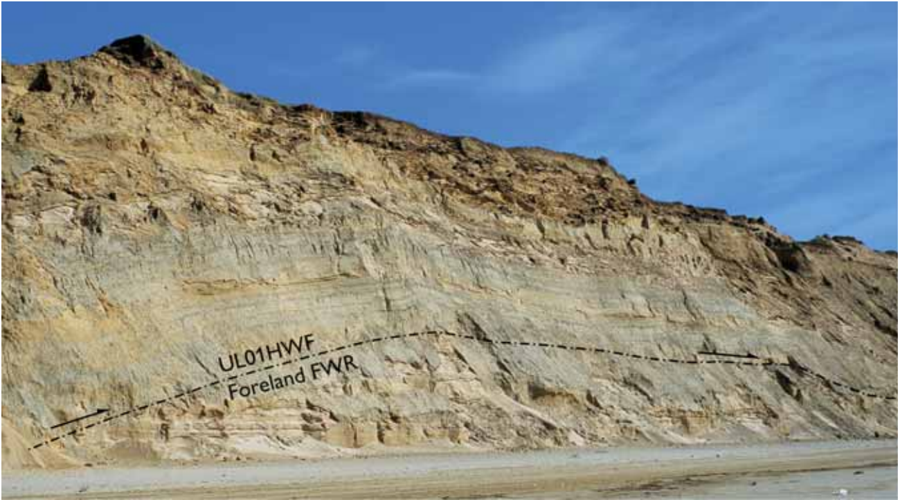
Fig. 43. The upper footwall ramp of the foreland (Foreland FWR) along which the UL01 thrust fault propagated ( UL01HWF : Ulstrup thrust sheet 01 hanging-wall flat), and from where it continued for more than 300 m over the footwall flat of the foreland. The cliff section is 25 m high and south is to the right. Photograph: May 1998.
