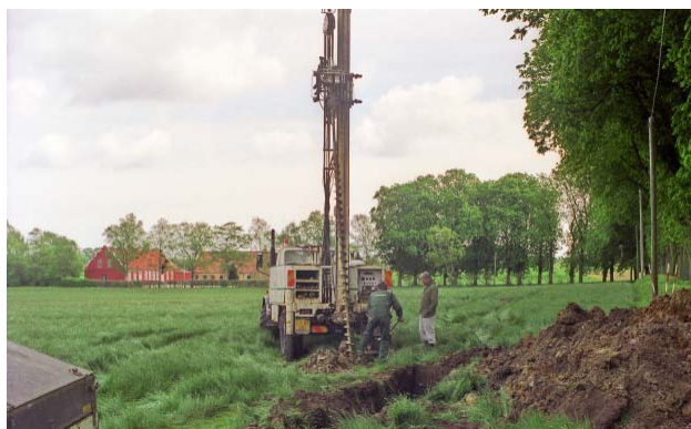
Fig. 2. Field investigations at the Lundeberg locality. Drilling close to the excavated trench.
