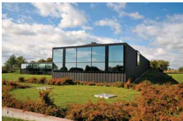
A modern Danish waterwork from Østerby, eastern Jylland.
